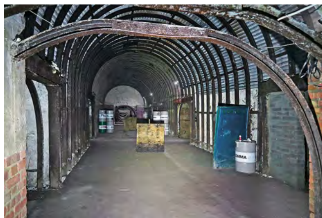
Former Ops Room deep beneath Fort Southwick with later airsoft barriers. The mixed construction of steel, brick and concrete can be seen. Traces of original dividing walls remain on the floor. Compare with the front cover picture from 2004 where the room is bare.
